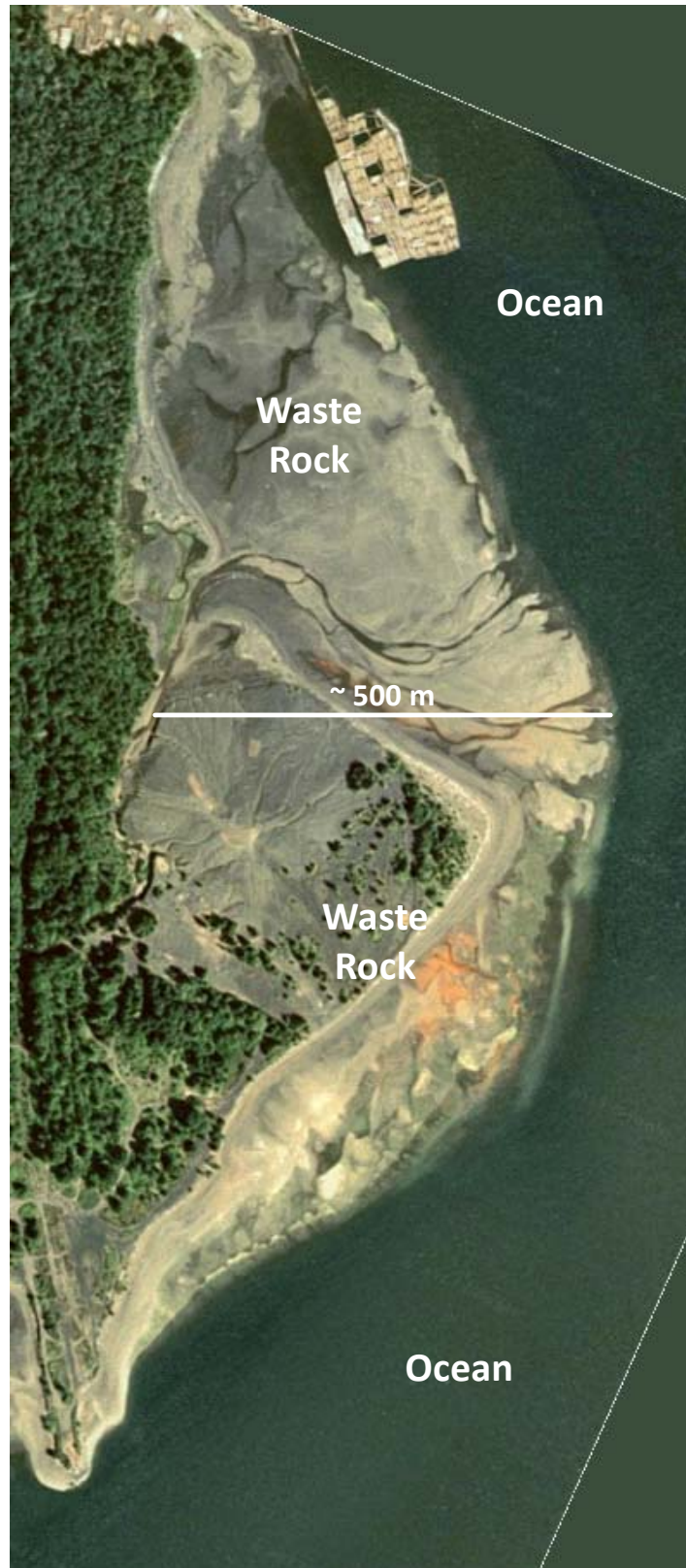
Photo 2-1. Air photograph of the coastal waste-rock pile.
