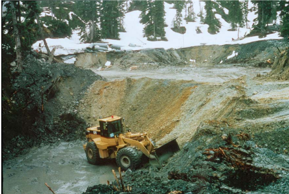
Figure 1-1. Photograph of the ongoing excavation of the ARD-releasing waste-rock pile at the Eskay Creek Minesite.
